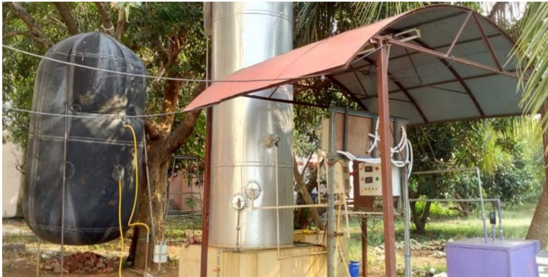
Fig.1 Layout of BENAKA-MVGR Biogas Plant
