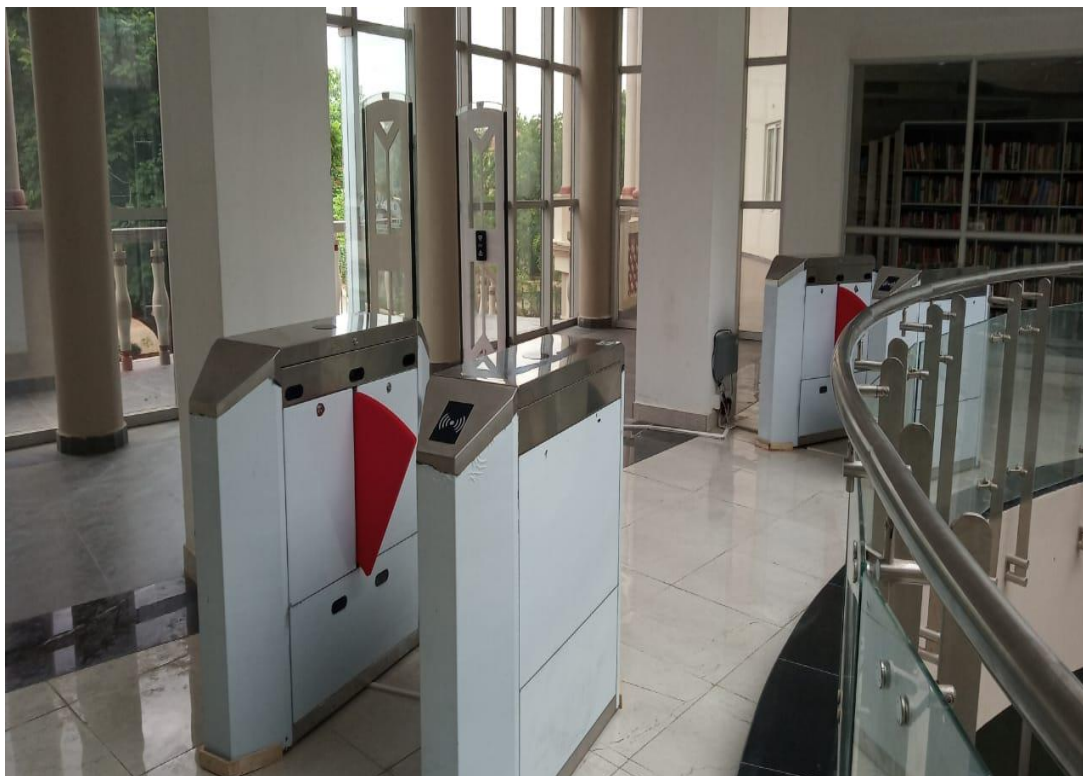
Flap Barriers (For entry and exit to the library)
