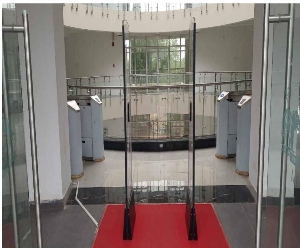
RFID Check gate (Security for library materials)
